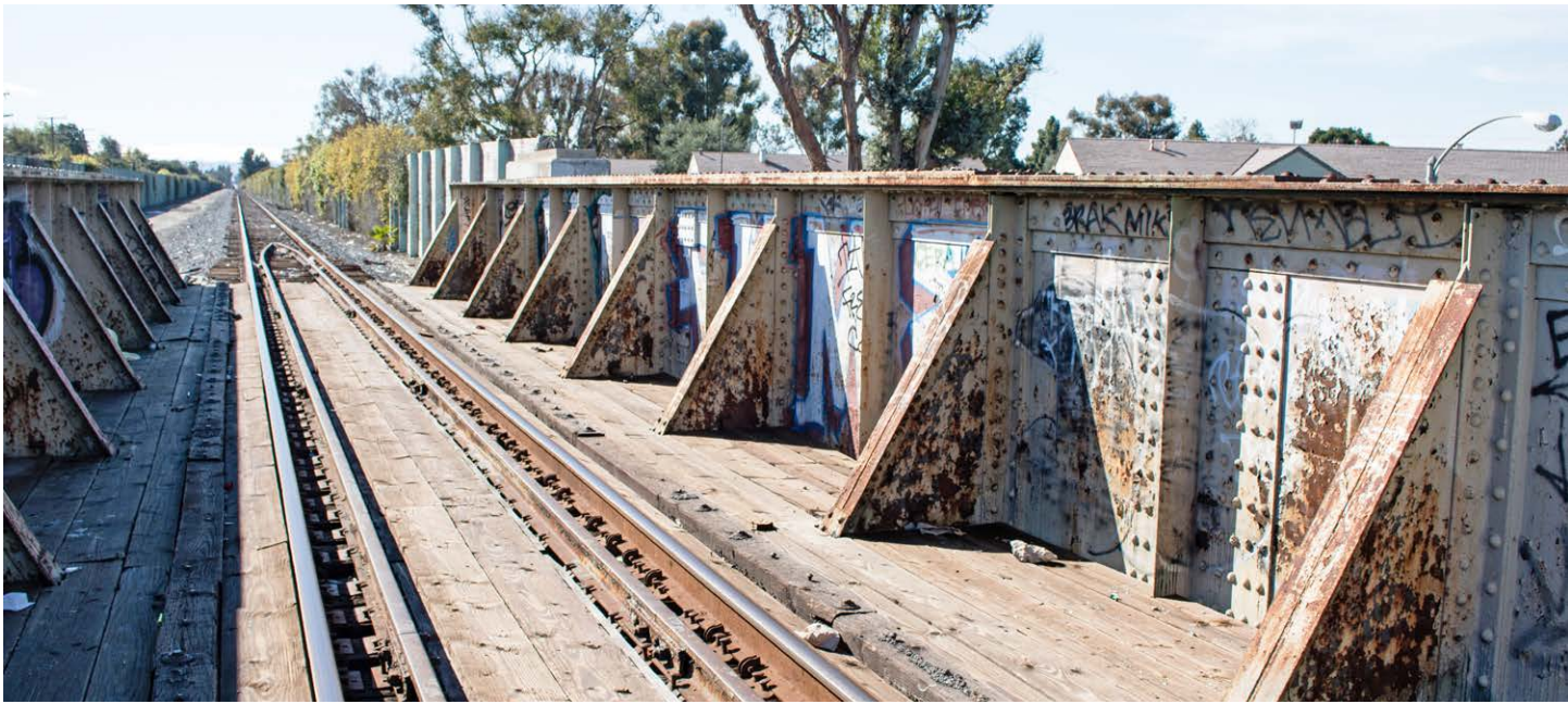
Above. Barriers Along the Railroad Corridor
