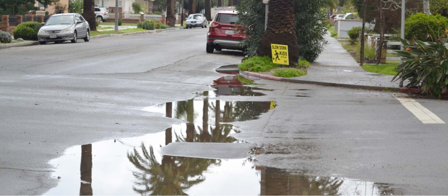
Above. Localized Flooding
