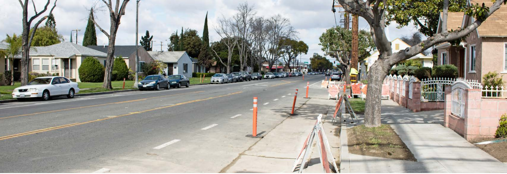
Above. Orange Avenue Bike Lane Construction
