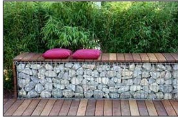
Gabion bench Gabion benches with wooden seat and wooden back will be constructed by the students and the community. The benches will also feature a planter bed serving as a table by barrier. Stone came out as one of the preferred materials from the community and the uneven surface makes it less vulnerable to vandalism and easy to maintain.
