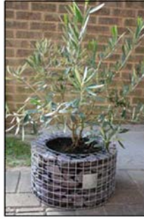
Gabion planter Circular gabion planters will be constructed by the students and the community. These planters will act as a safety buffer from the traffic on the street as well as act as an edge of the parklet.
