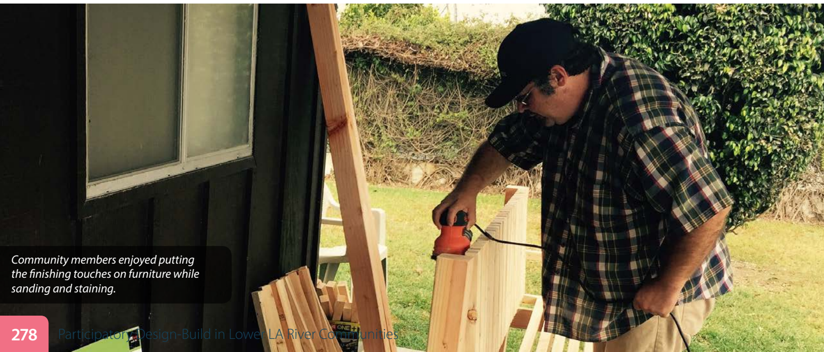
The project team found building prototypes in the shop helped prepare for community work days.
